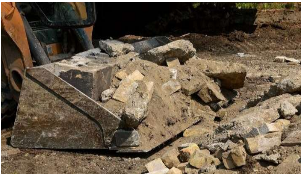
Fig-21 Cleanup excavator
