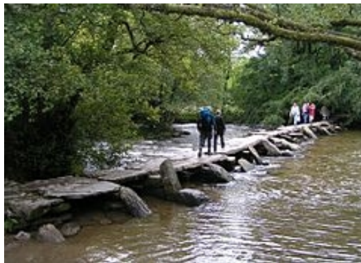
Fig-3 Clapper bridge
