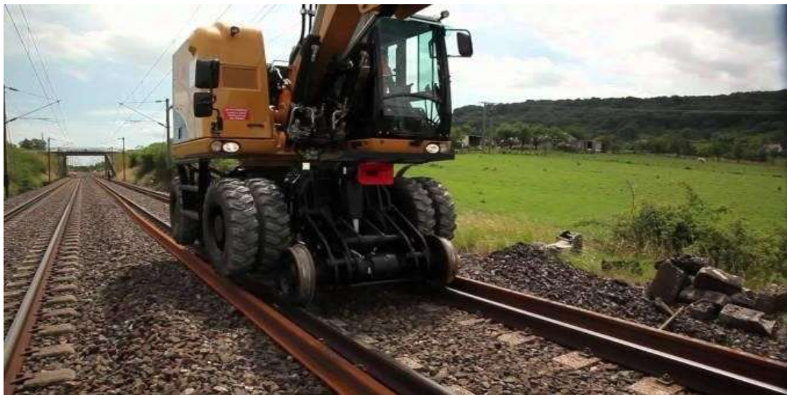
Fig-18 Barge rail mounted
