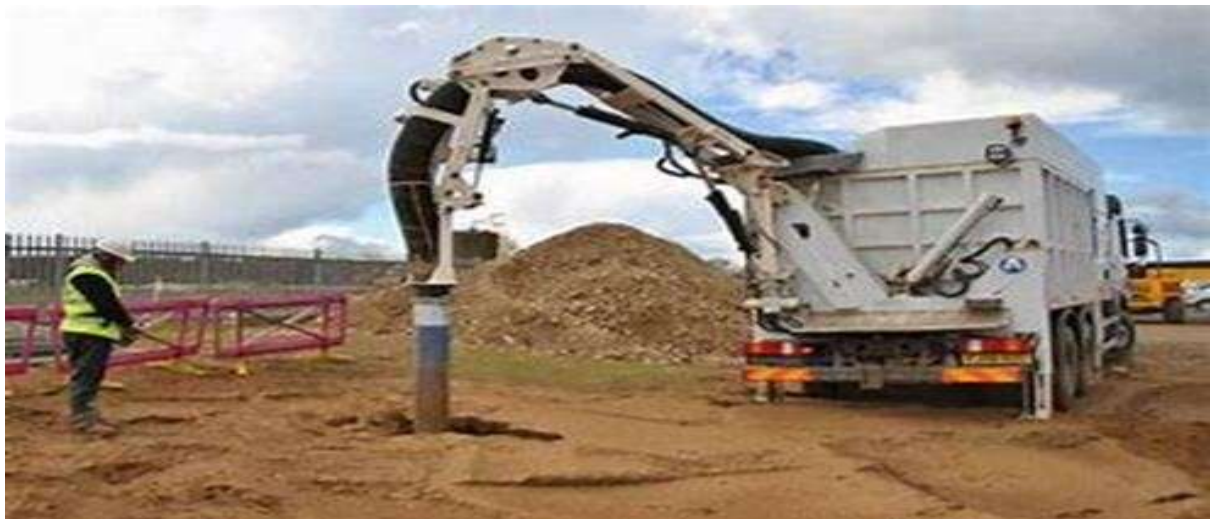
Fig-4 Suction excavators
