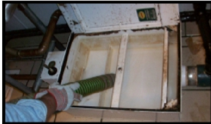
Fig5. Cleaning of hydromechanical grease interceptor
