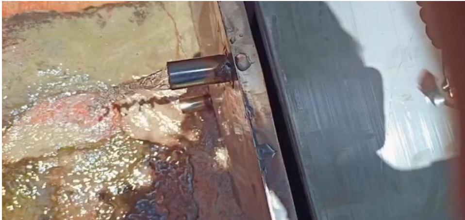
Figure 24 – Automatic separation of water from fogs and food particles.
