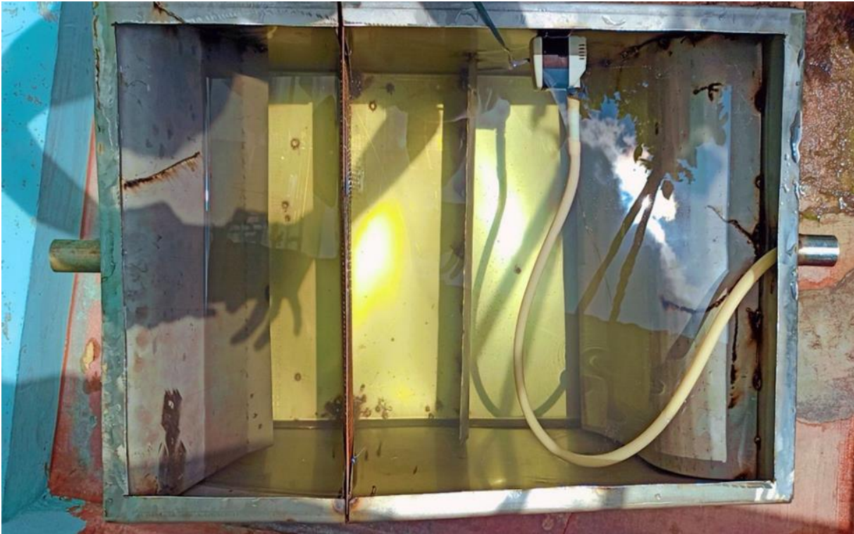
Figure 21 – Installing pump for automatic removal of grease.
