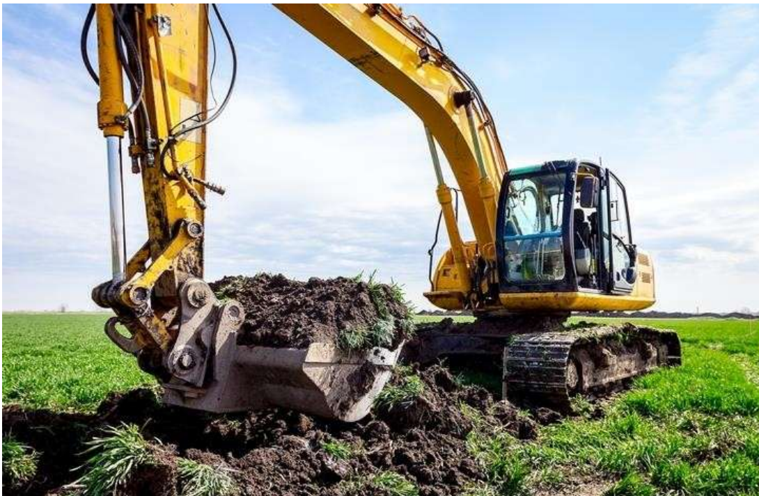
Fig-19 Digging excavator bucket
