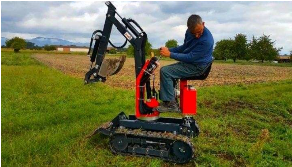
Fig-17 Self Propelled excavator
