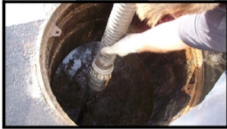
Fig7. Cleaning of Gravity grease interceptor
