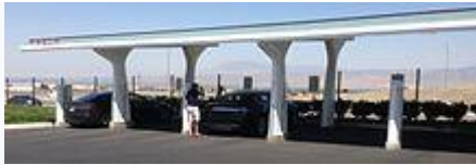
Fig:2.4 Tesla Supercharger rapid charging station in Tejon, California. The rooftop of the carport has a solar collector manufactured by SolarCity feeding energy into the grid.
