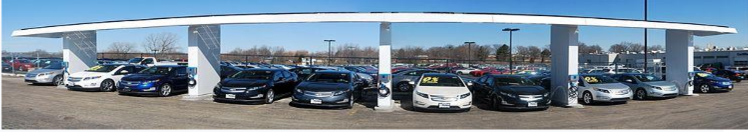
Fig:2.9 Several Chevrolet Volts at a charging station powered with solar panels in Frankfort, Illinois.
