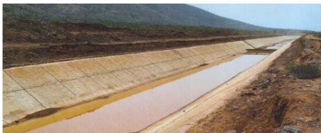
Figure 3.10: Right main Canal
