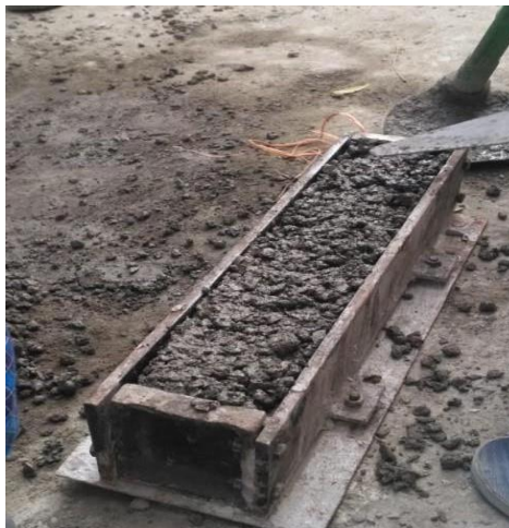
Figure 10: casting of prisms
