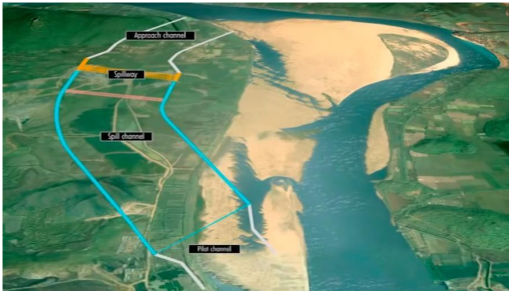
Figure 3.3: Representative image of Spill way (Orange coloured mark)
