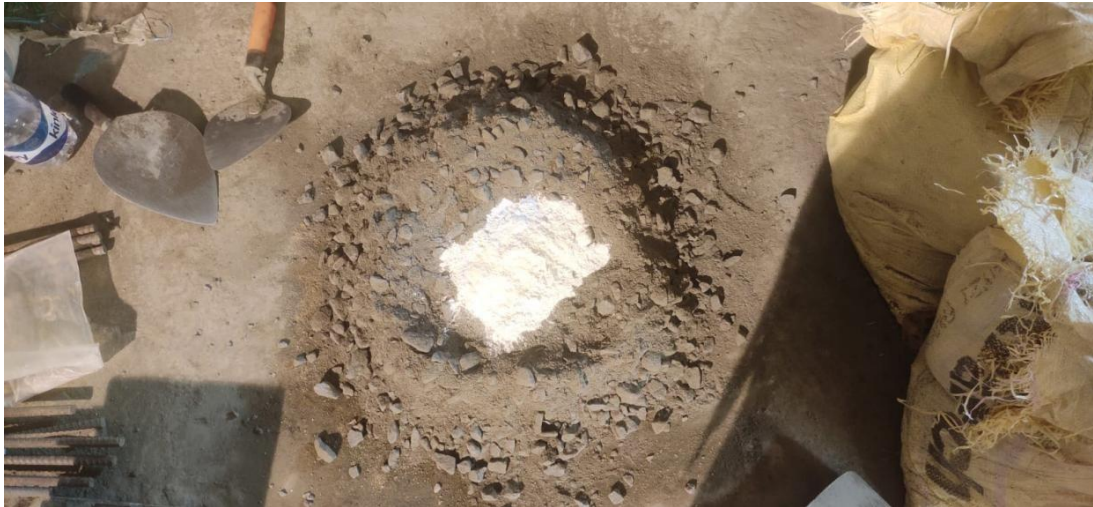
FIG 4.0 MIXING OF CONCRETE
