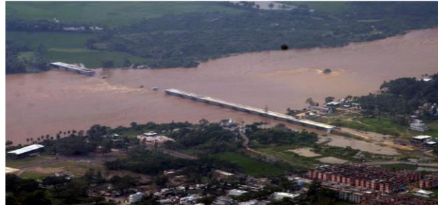
FIG 1.2: Disaster due to flood
