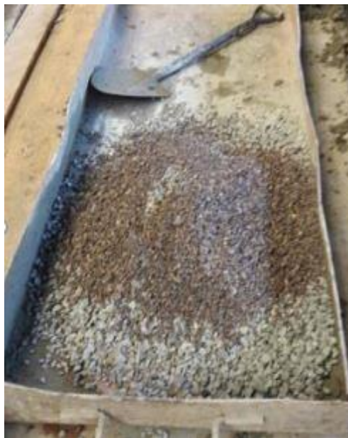
Figure 3-7: Tray used for the mixing of concrete.
