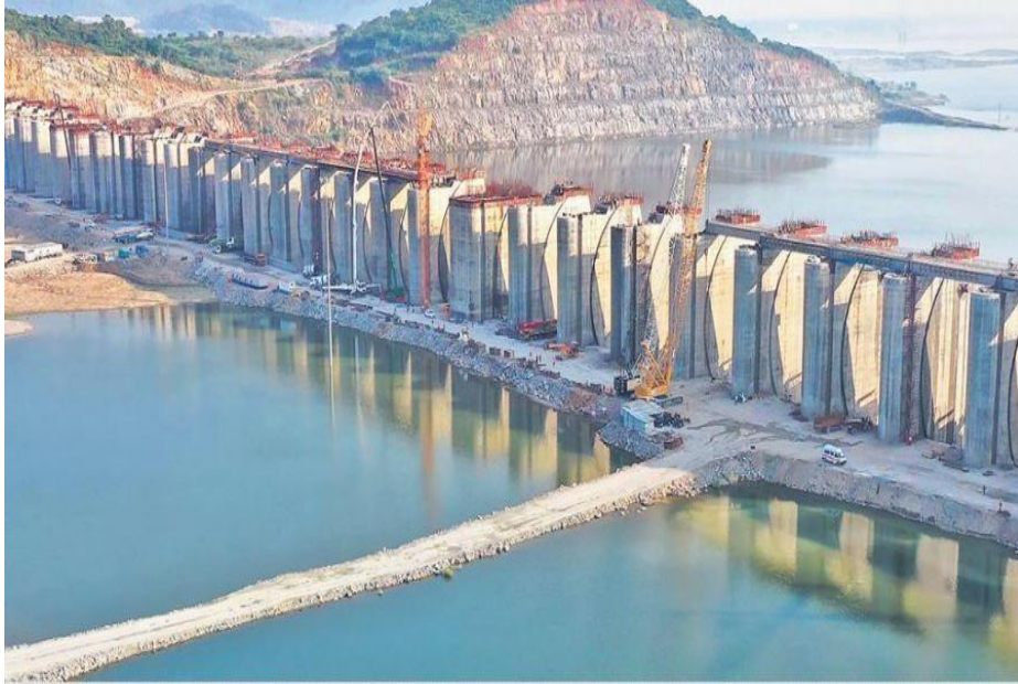
Figure 3.4: Image of Earth cum Rockfill Dam (Polavaram Dam) from Google application
