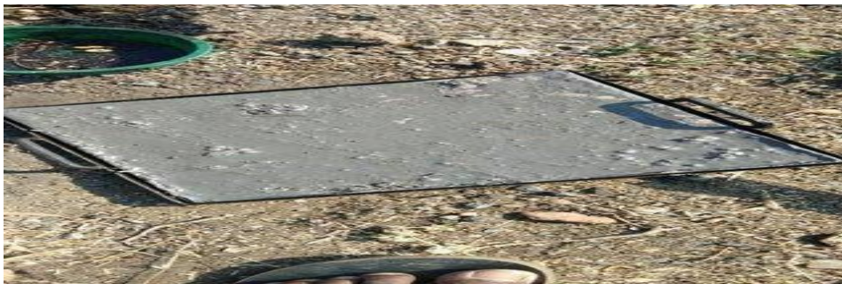
Figure 8- Completely prepared mould.
